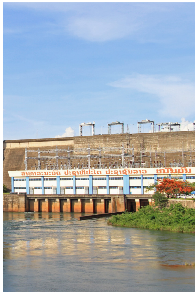
Nam Ngum hydroelectric power station in Laos. Source: MatyasRehak/Shutterstock
