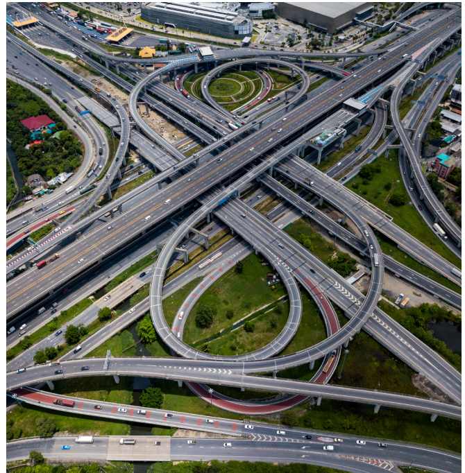
Aerial view of highway junctions in Bangkok, Thailand. Source: Travel man/Shutterstock
